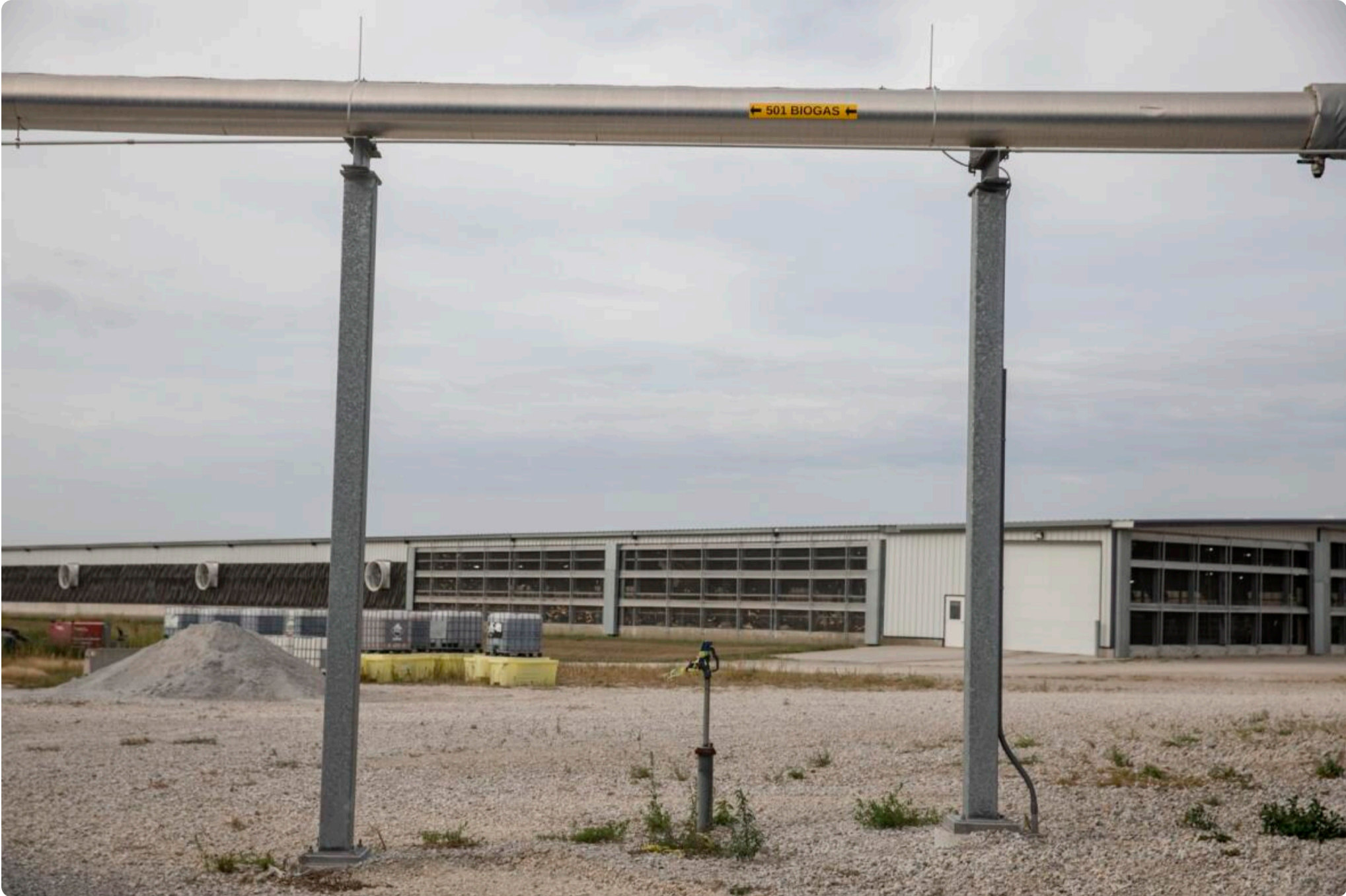
Dairy barns and a gas pipeline at the Marshall Ridge Renewable Energy Center in State Center on Sept. 18. The facility's three anaerobic manure digesters extract methane from dairy cow manure. The Marshall Ridge project produces 250 and 325 MMBTU of renewable natural gas per day. (Nick Rohlman/The Gazette)
