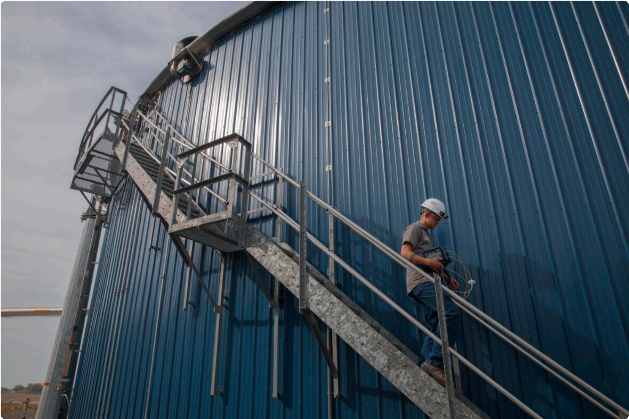
Technician Blake Iske descends a set of stairs after taking a sample measurement at the Marshall Ridge Renewable Energy Center in State Center on Sept. 18. The facility's three anaerobic manure digesters extract methane from dairy cow manure. (Nick Rohlman/The Gazette)
